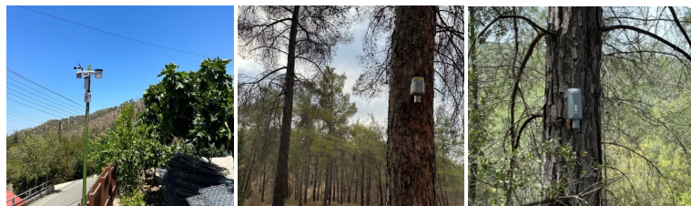
Figure 3. Installations (Weather Station, EM500, SenseCAP S2103).
