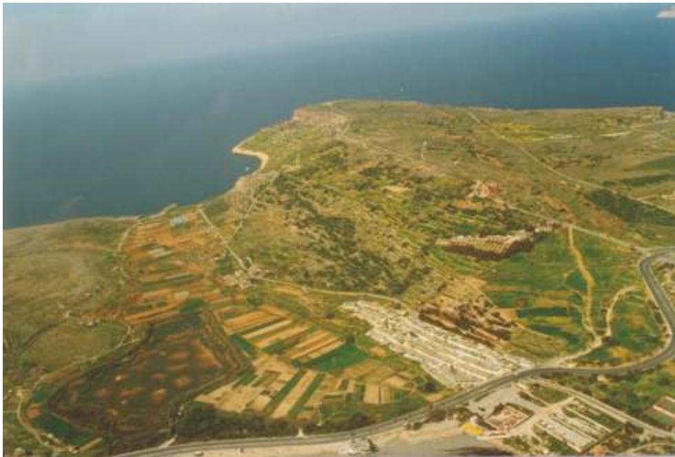
Fig. 2. An aerial view of the area: the Ghadira wetland is visible in the lower part
