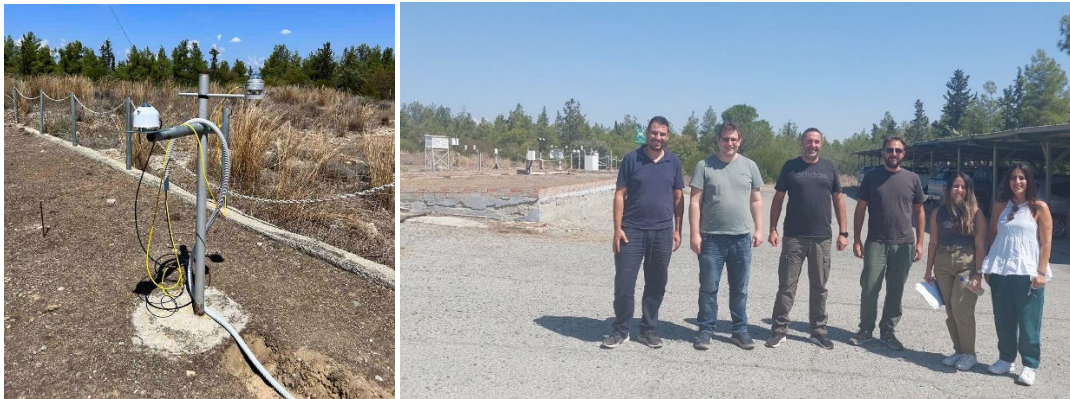
Figure 32 Installation of Solar Radiation equipment
