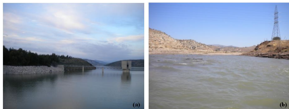
Figure 3. Picture of Asprokremmos focused in the (a) Outlet Area & (b) Inlet Area of the Dam.
