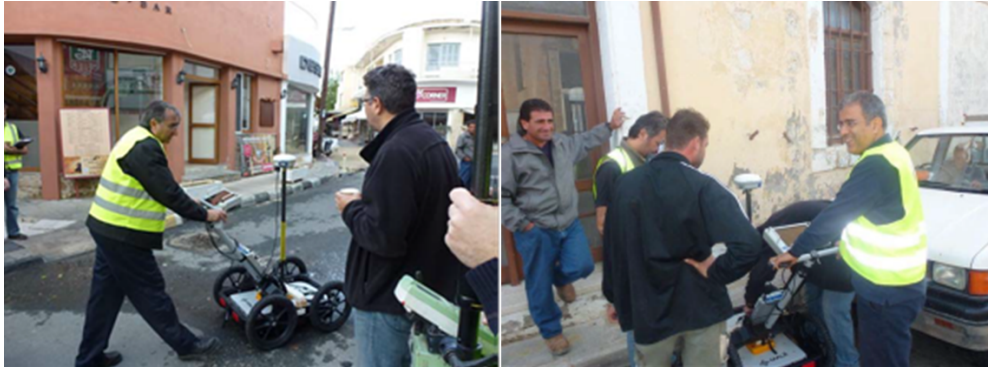
Figure 2. Geo-radar Scanning of the Paphos water utility network
