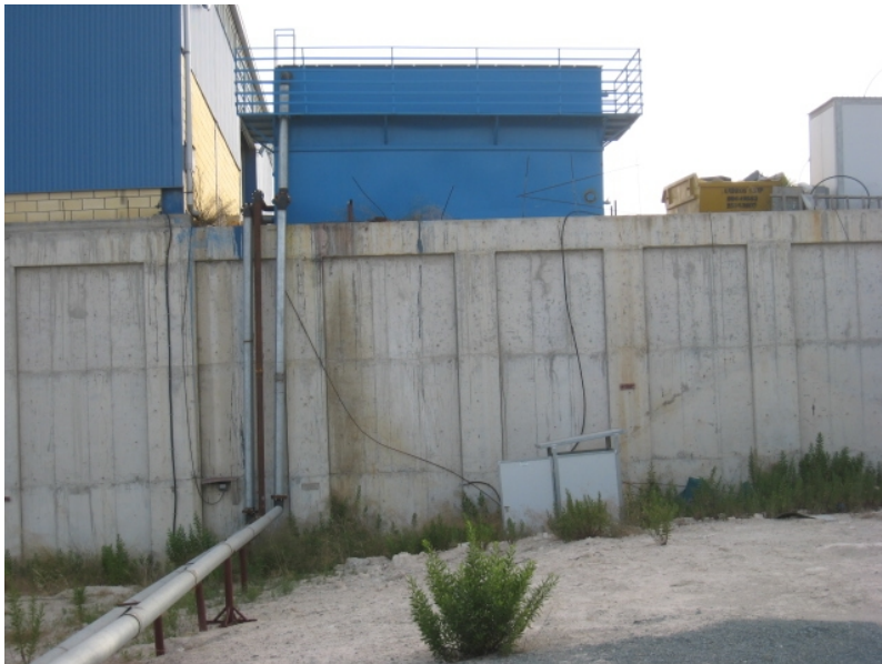
Figure 11. Constant head tank
