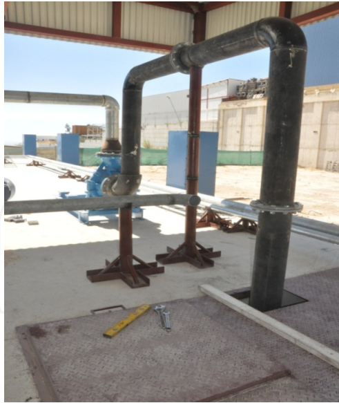
Figure 8. Pipe network during construction
