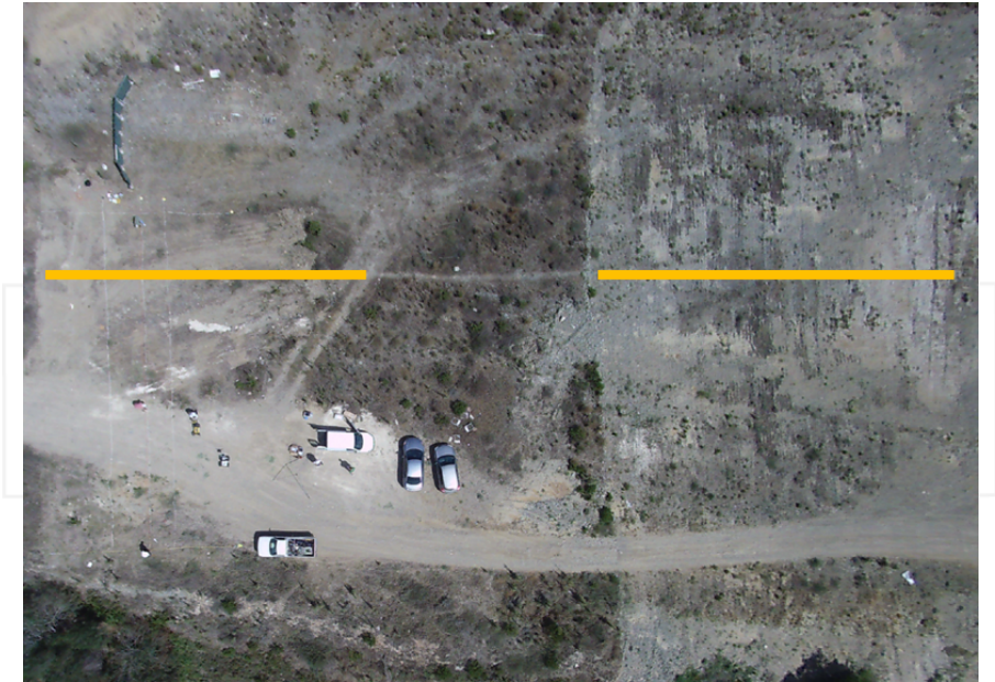
Figure 5. Lakatameia underground pipeline as observed from UAV
