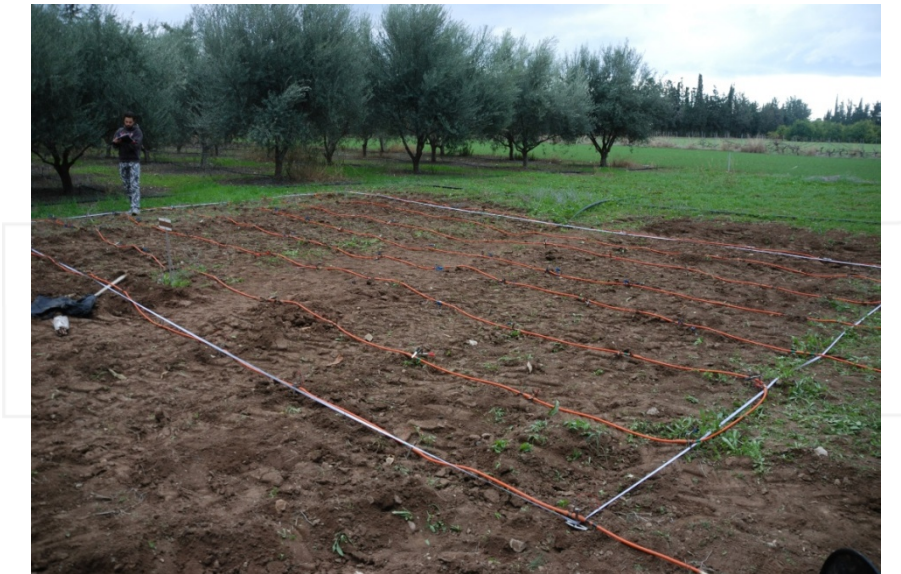
Figure 1. Area of interest. A pipeline was buried at a depth of approximately 1 meter.
