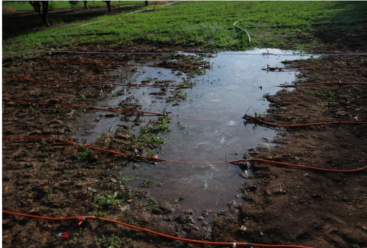
Figure 2. Leakage as observed from the surface
