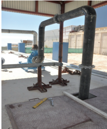
Figure 8. Pipe network during construction
