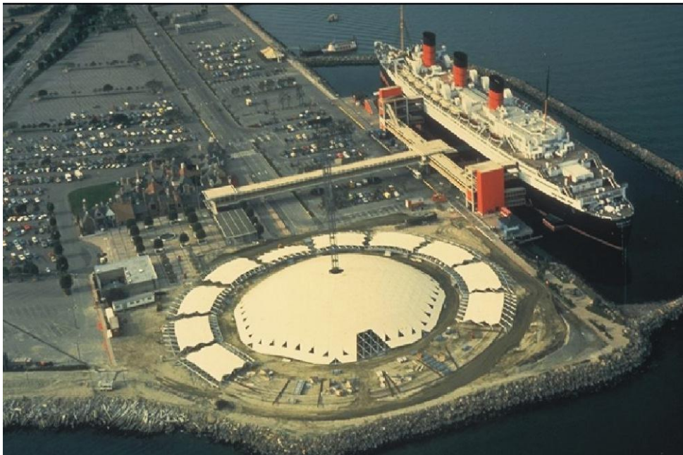
Εικόνα 10: The “Spruce Goose” dome during erection (Long Beach, California)
