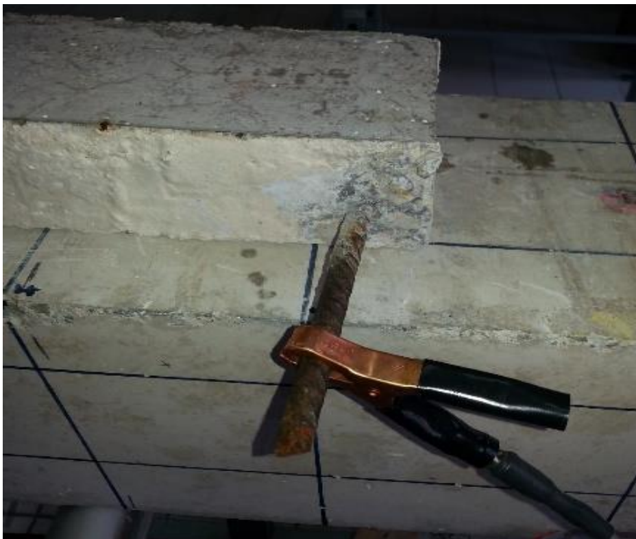
Figure 13: Attached cable to the exposed steel to create a circuit
