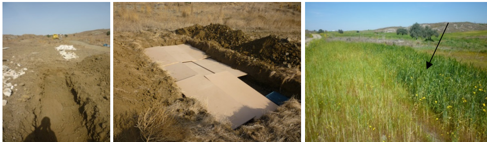
Figure 1. Photos during the construction of the test field in the Alampra area. The formation of crop marks is indicated with an arrow in the right photo (34°58'46.22"N, 33°23'2.48"E).
