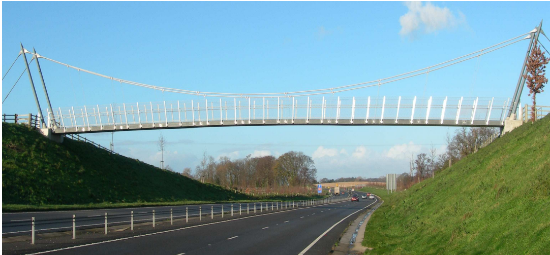
Figure 1. View of the completed Wilcott footbridge
