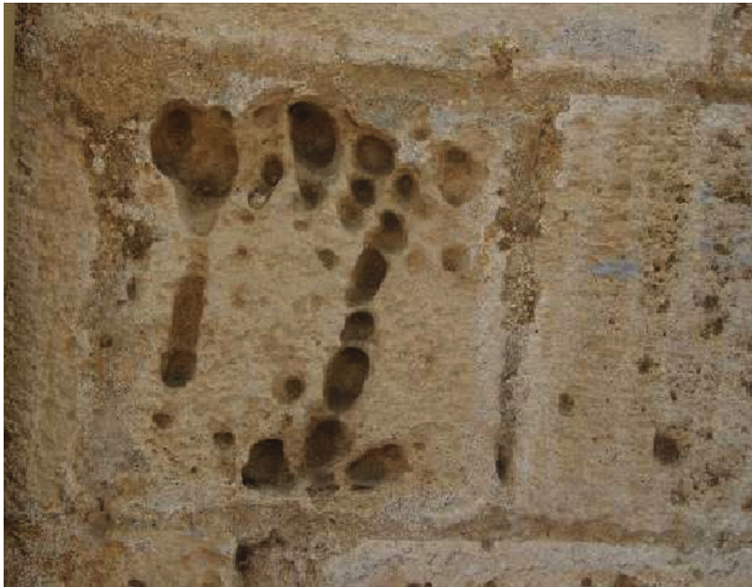
Figure 20: Honeycomb formation on the surface of the limestone block.
