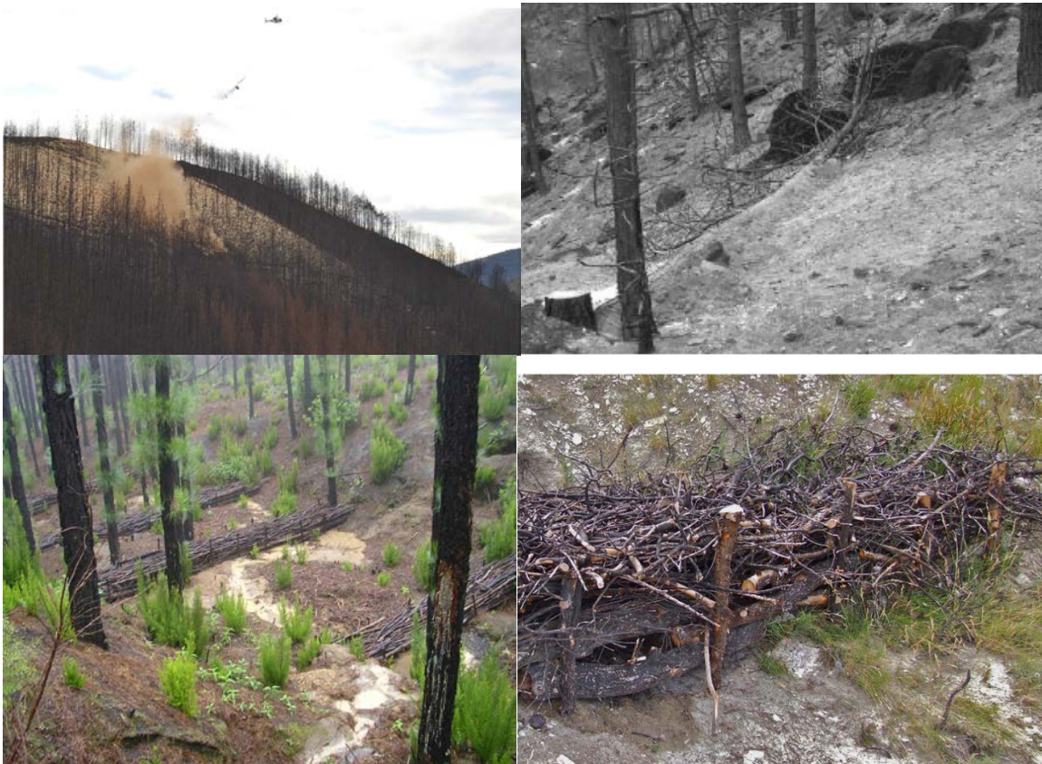
Examples of PEFTs, including (in order of appearance): Heli-mulching operations, contour-felled log, in-channel check dams (wooden); hillslope log debris dam 4 .
