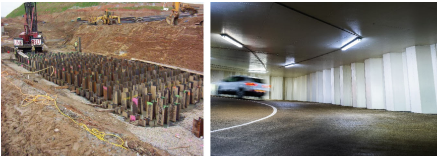
Fig. 5.4 Steel as a reclaimable foundation element
