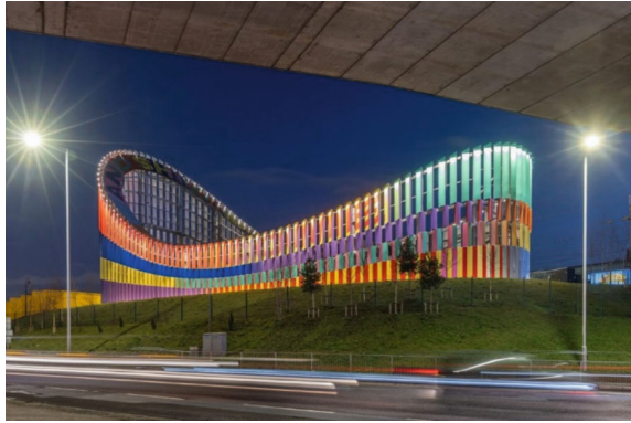
Fig. 5.5 Brent Cross Town primary substation [43]
