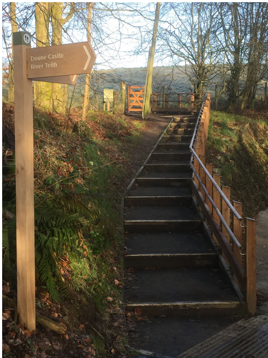
Fig. 7 New stepped ramp leading from Doune Castle past the Roman Fort. © Historic Environment Scotland
