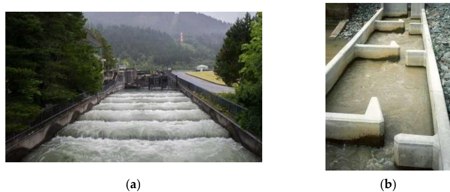
Figure 3. (a) Pool-and-weir fish ladder, (b) vertical-slot fish ladder.
