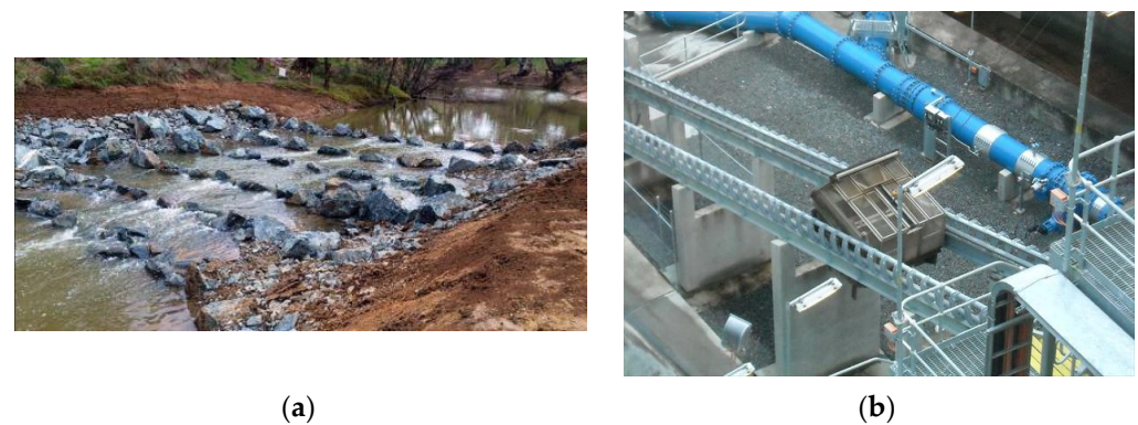
Figure 4. (a) Rock-ramp fishway, (b) fish lift at Tallowa dam.
