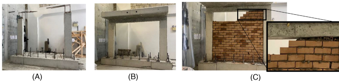
FIGURE 3 Construction of masonry-infilled RC frame (A) placement of precast RC columns and foundation RC beam, (B) construction of RC T-section beam, and (C) building of masonry infill wall with detail of the last row of bricks.
