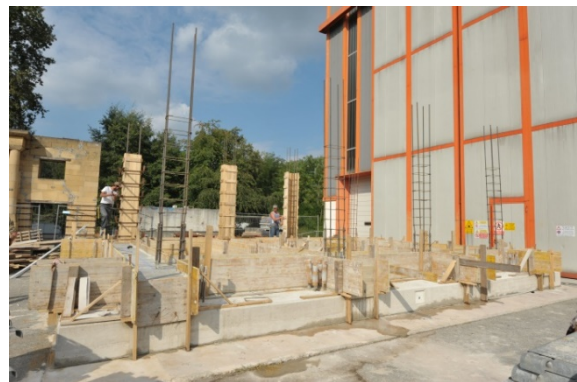
Figure 4.2 Foundation slab with column reinforcement
