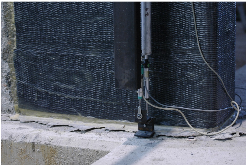
Figure 8.4 Position 7: Crack opens at the bottom of the column - wall
