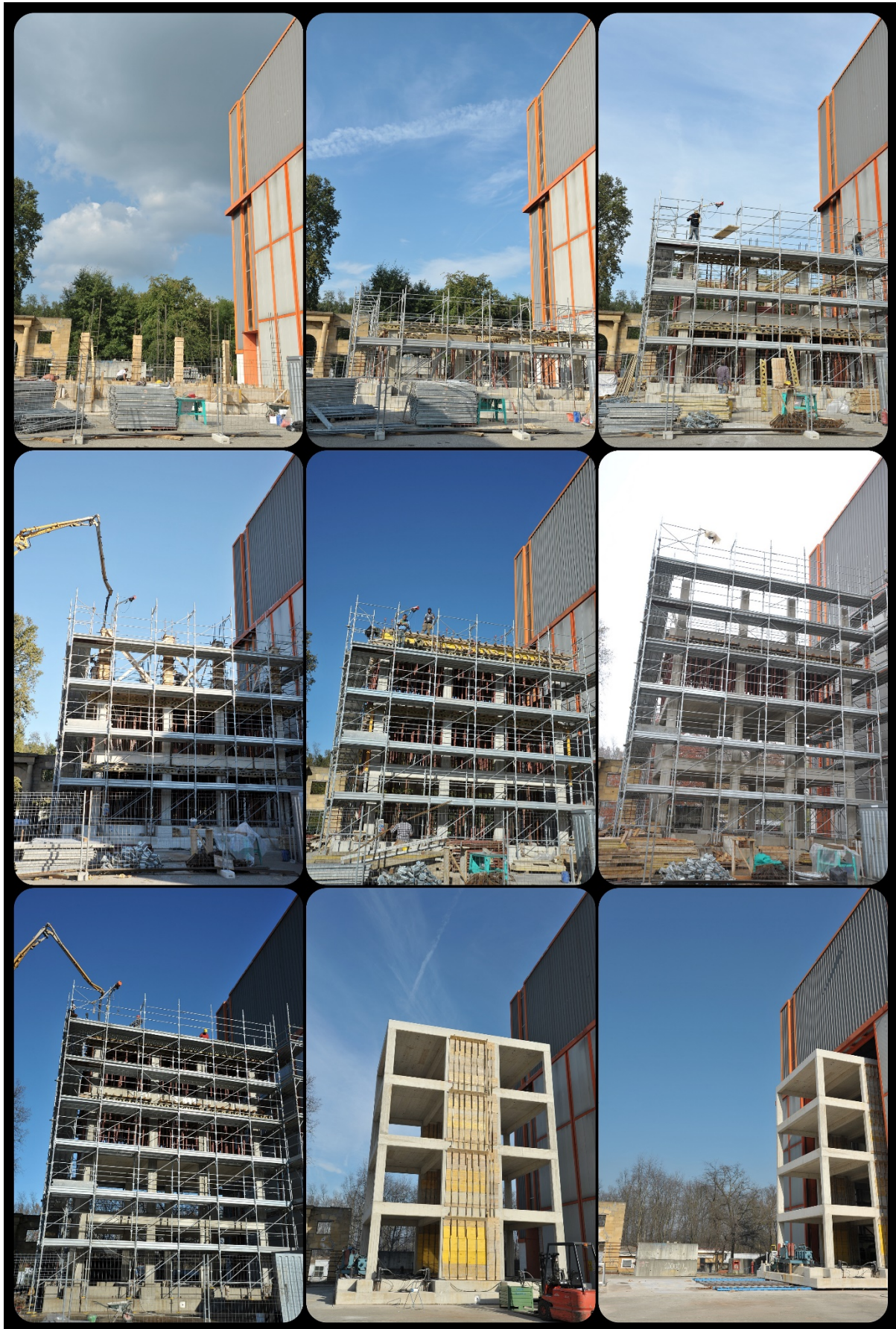
Figure 17 Construction phases of the SERFIN structure
