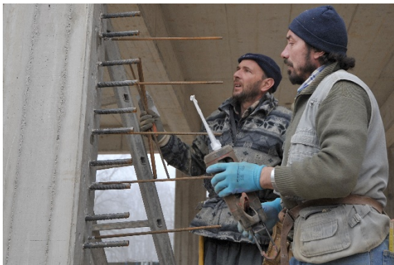
Figure 4.15 Installation of dowels and starter bars
