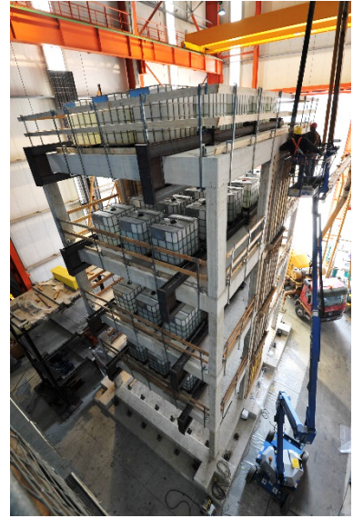
Figure 5.3 Vertically loaded structure; infill walls pouring
