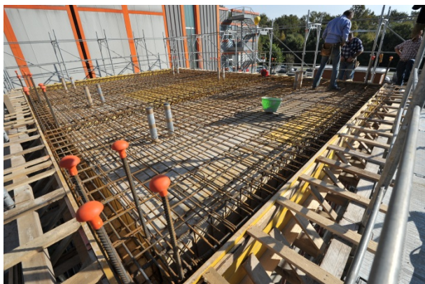
Figure 4.7 Slab reinforcement
