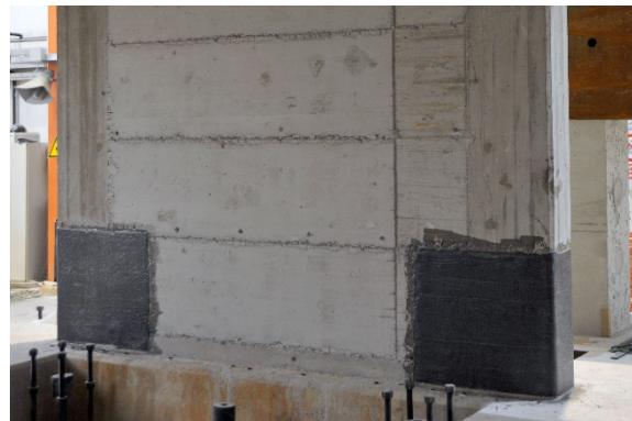
Figure 4.16 CFRP reinforcement jacket of the ground columns in the north frame
