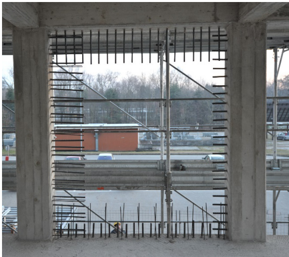
Figure 4.13 Dowels and starter bars
