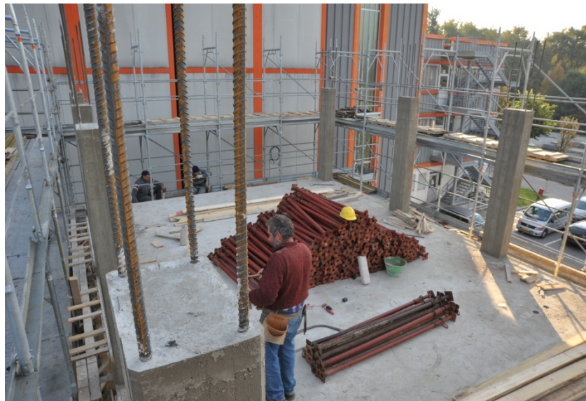
Figure 4.6 Columns in the third storey
