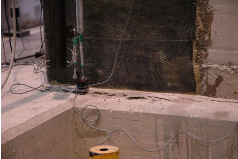
Figure 8.2 Position 6: Crack opens at the bottom of the column - wall
