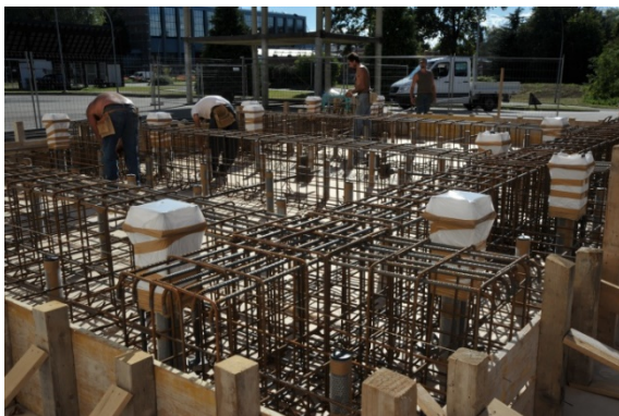
Figure 4.1 Foundation slab reinforcement
