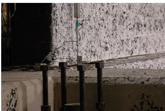
Figure 8.12 Position 2: Crack opened under the CFRP jacket
