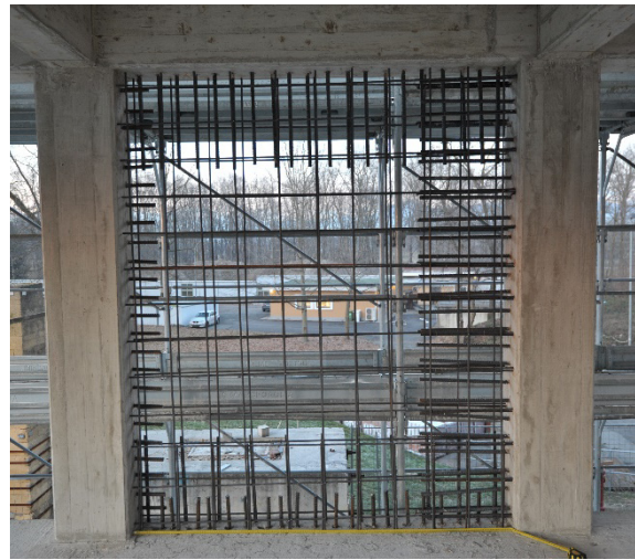
Figure 4.14 Dowels, starter bars and web reinf.
