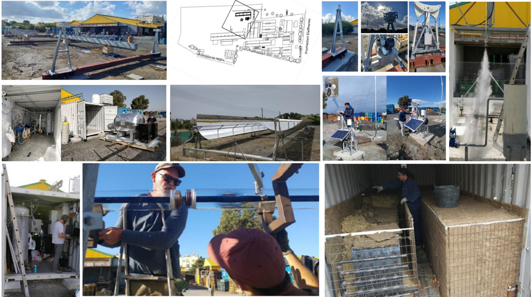
Figure 45: Photos of installation procedure and first operation tests.
