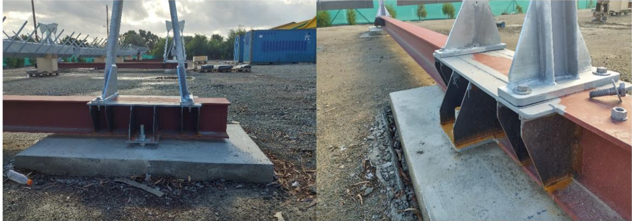
Figure 80: I-beams connected to the concrete infrastructure.
