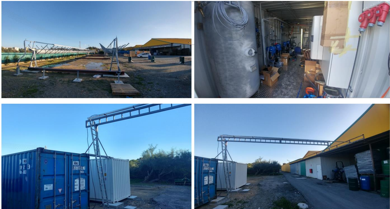
Figure 88: Supply of the produced steam with the industry's steam distribution system.
