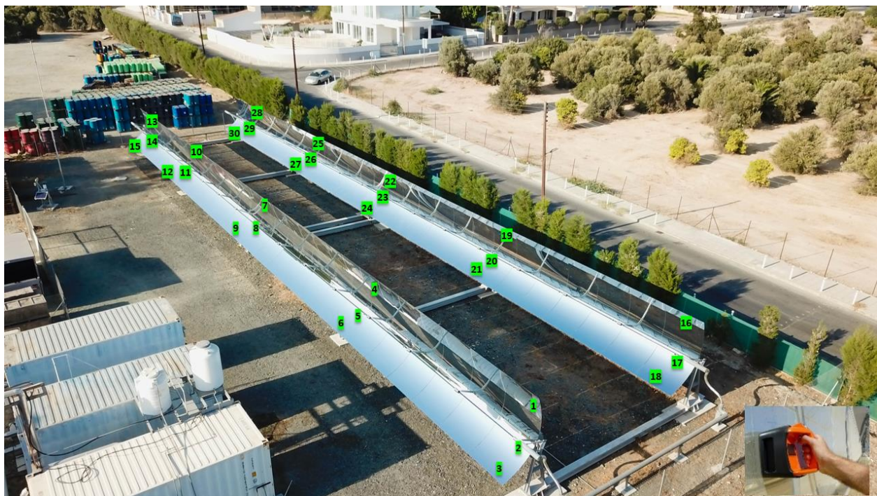
Figure 65: Reflectivity measurement points along the collector length.
