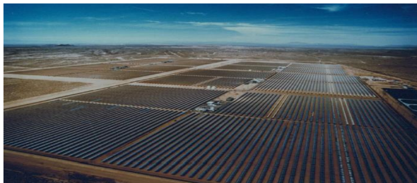
Figure 5: SEGS Thermal plant in California (Sandia National Laboratories: Exceptional Service in the National Interest, 2020).
