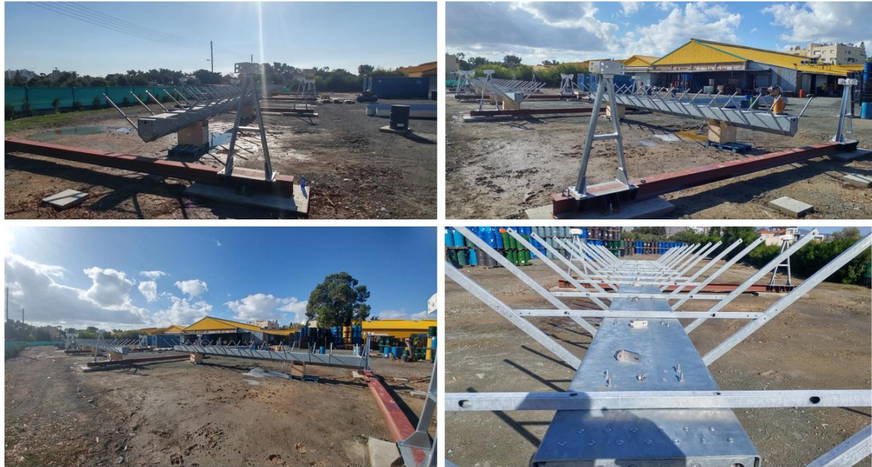
Figure 81: Collectors assembled
