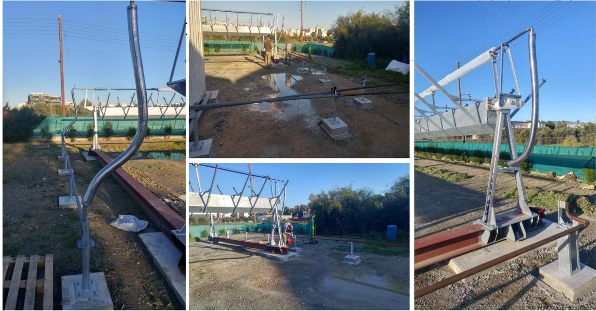
Figure 87: Connection of the PTC receiver tube with distribution pipe via a flexible connector.
