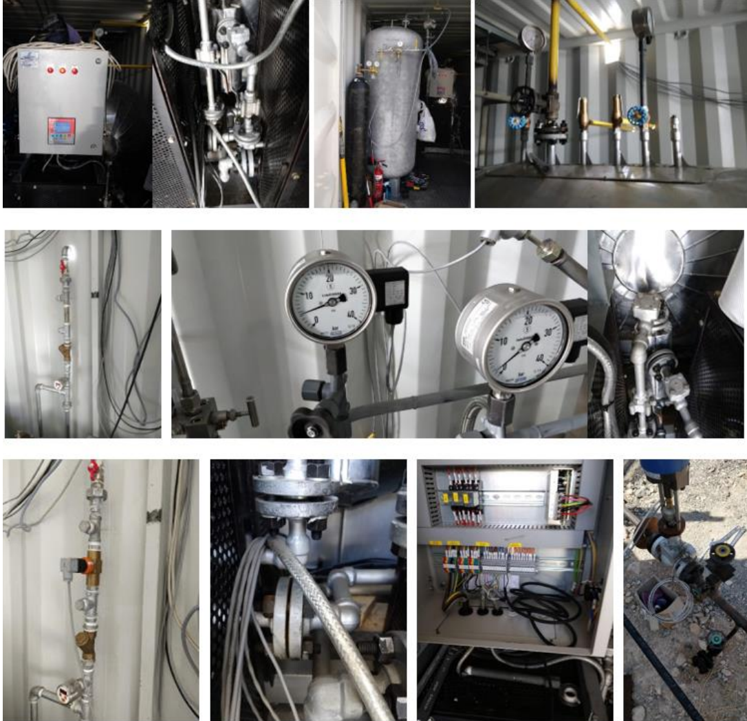
Figure 97: Elimination of leakages and installation of instruments and alarms.
