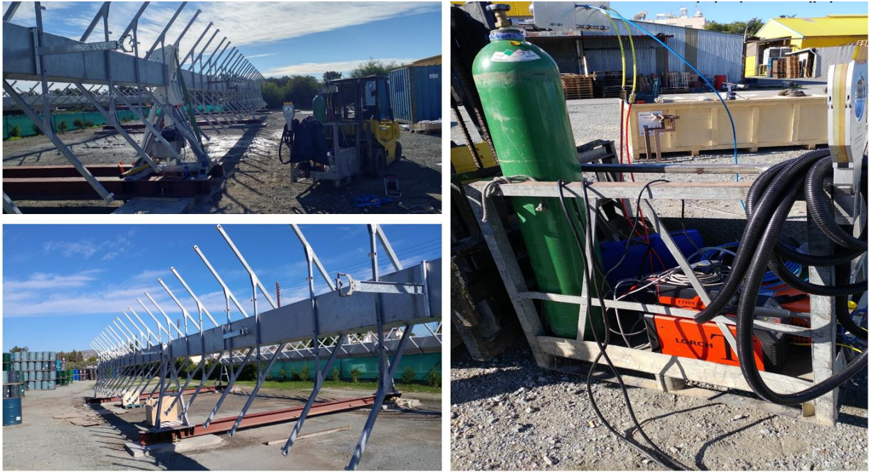
Figure 84: Preparation of the collectors for a ticking welding.
