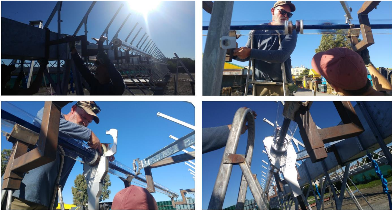
Figure 85: The welding procedure.
