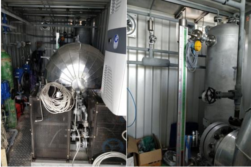
Figure 93: Steam Generator and parts installed.
