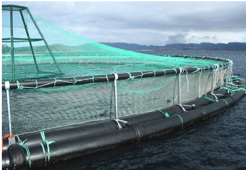
Fig. 1 Floating fish farm with circular plastic collar consisting of two concentric rings. The photo is taken from [Faltinsen (2011)]. (Photo: SINTEF Fisheries and Aquaculture)
