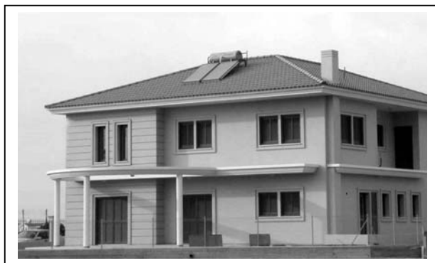
Fig. 4 Pressurised solar water heater installed on an inclined roof.
