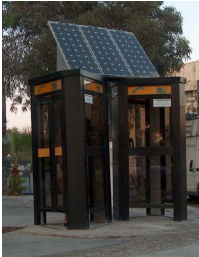
Fig. 9 Telephone booth powered by PV
