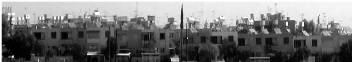
Fig. 1 Practically every house in Cyprus is equipped with a solar water heater.
