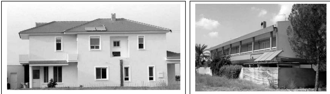
(a) Installation on an inclined roof of proper inclination (b) Installation detached from the house. Fig. 7 Applications of force circulation type solar water heaters.
