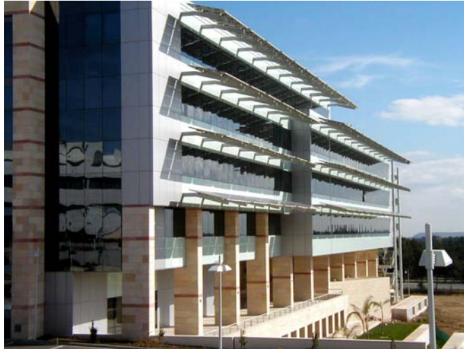
Fig. 10 EAC Headquarters PV shading system
