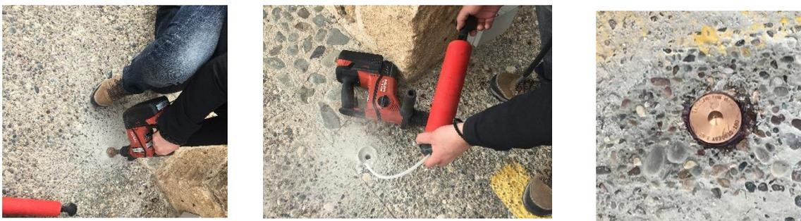
**Figure 3.** Installation of TG benchmarks using high-quality levelling markers.
