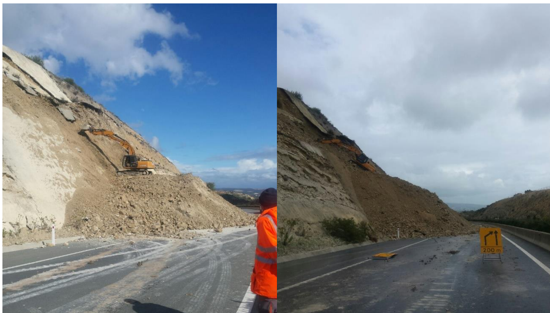
Figure 124: Rehabilitation works at the landslide area – Pissouri (Geological Survey Department)
