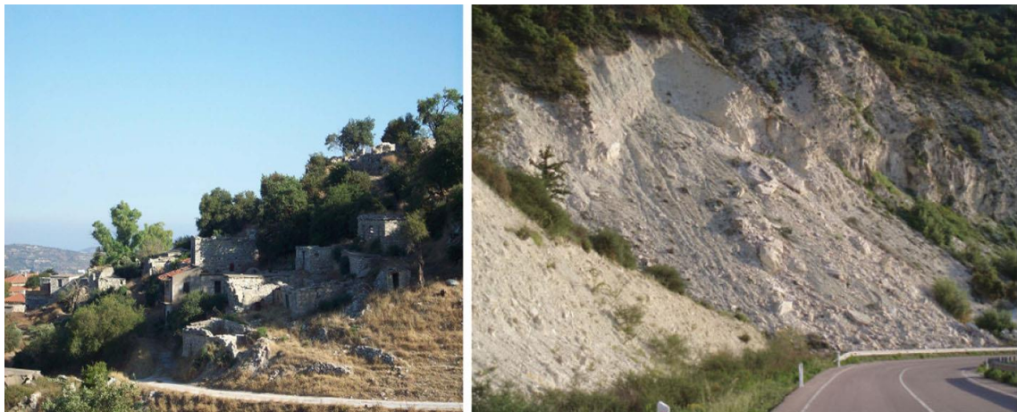
Figure 19: The evacuated village of Statos (left). Rockslide in chalk across a roadcut (right)
