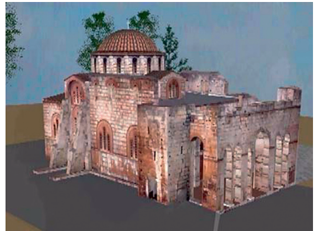
Fig. 2. Textured 3D model of the external of the Katholikon of Dafni monastery, produced by the combined use of surveying and photogrammetric techniques.
