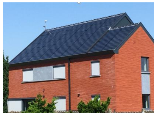
Figure 12: The 57 RS modules on the roof of the demonstration building.
