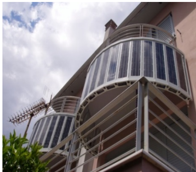
Fig. 1 Balconies PV Subsystem
