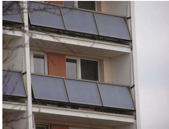
Solar collectors act as balcony railings of the building, Beijing, China
