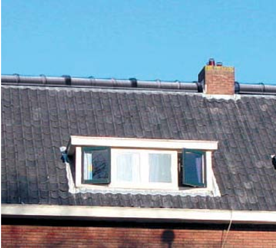
Eco-Nok roof integrated solar water heater, The Netherlands
