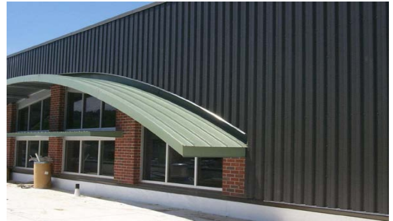
Rapid City Community Centers, SD, USA
