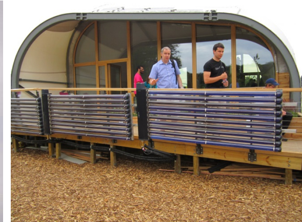
Solar collectors act as balcony railings of the building, Beijing, China
