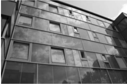
Figure 3. An indirect solar-comb construction BISTS.
