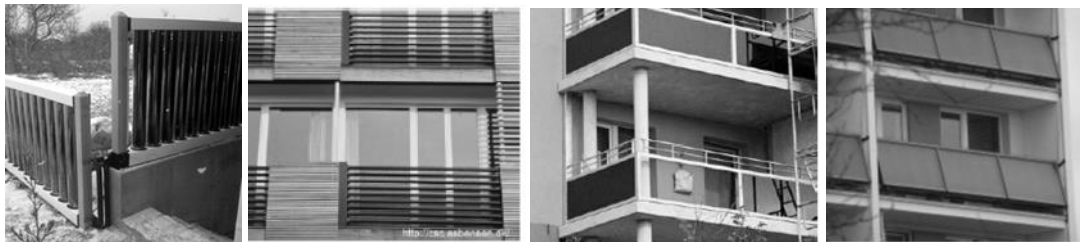
Figure 9. BISTS balustrade/railing feature.
