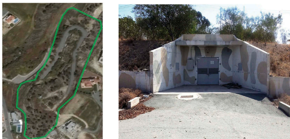
Figure 1. Overview of the study area (left); an example of a military bunker (right).
