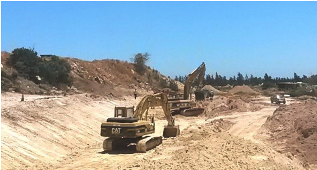
Figure 11: The construction site.
