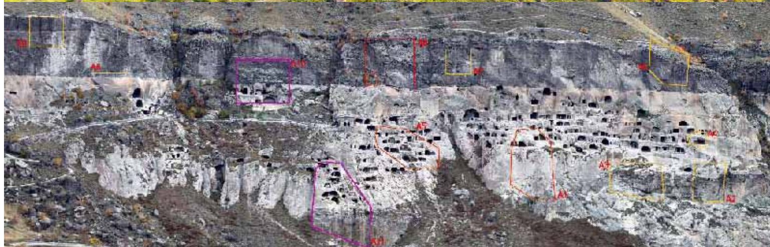
Unstable maps from the displacements maps obtained after two years of GBR monitoring
