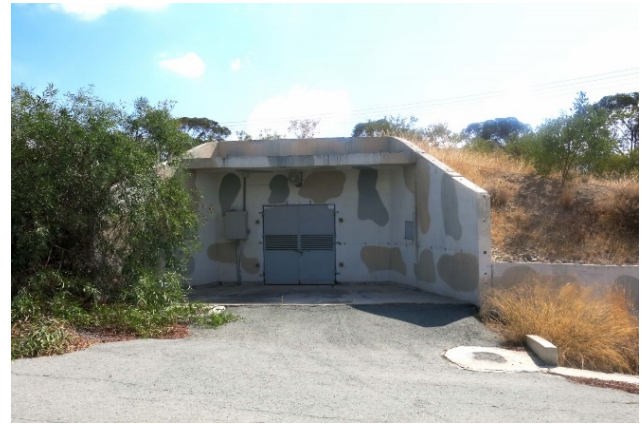
Figure 2. A military storage bunker.
