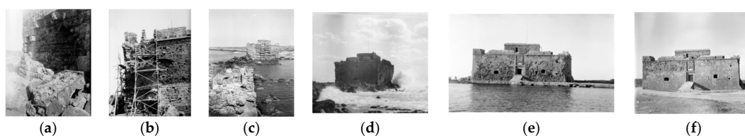
Figure 2. (from left to right): (a) Extended destruction of the external masonry wall (Archive of the Department of Antiquities of Cyprus, 1936); (b) Restoration works on the external north wall (Archive of the Department of Antiquities of Cyprus, 1939); (c) Conservation works on the south wall masonry (Archive of the Department of Antiquities of Cyprus, 1938); (d) The absence of water break infrastructure led to monument exposure, especially its western side (Archive of the Department of Antiquities of Cyprus, 1939); (e) East façade (Archive of the Department of Antiquities of Cyprus, 1939); (f) East façade (Archive of the Department of Antiquities of Cyprus, 1964).
