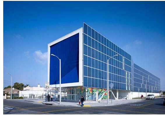
Figure 1.3. Photovoltaic panels on the building's facade.
