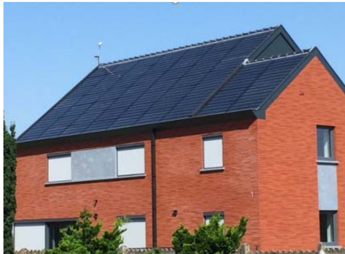
Figure 6.2. The 57 RS modules on the roof of the demonstration building.
