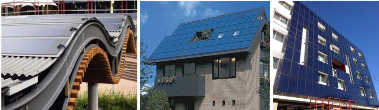
Figure 1.10. BIPV applications for solar heating.
