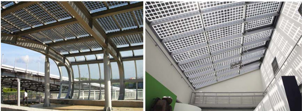
Figure 1.11. BIPV applications for natural lighting in buildings.
