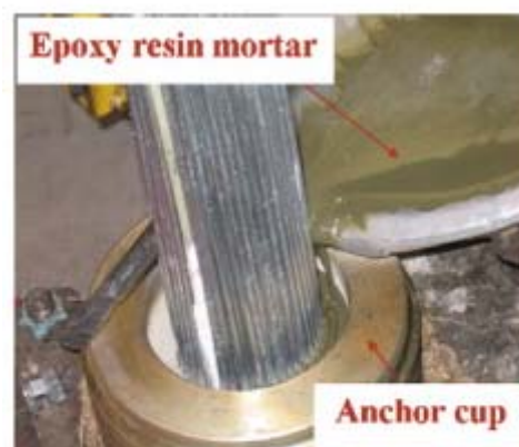
The anchor cup containing cable end, anchor and cover plates and epoxy resin mortar
