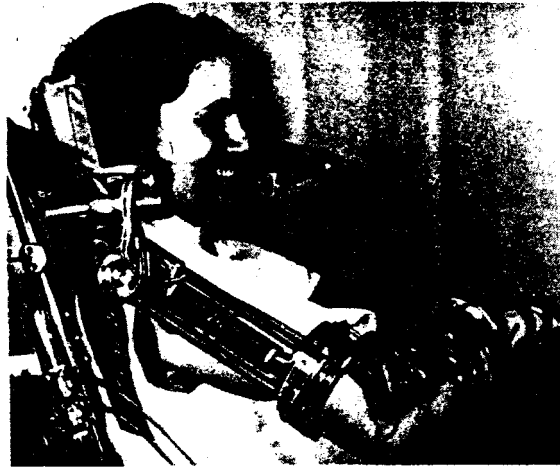
Fig. 1.5: An early wheelchair arm-aid operated by the handicapped person's tongue
