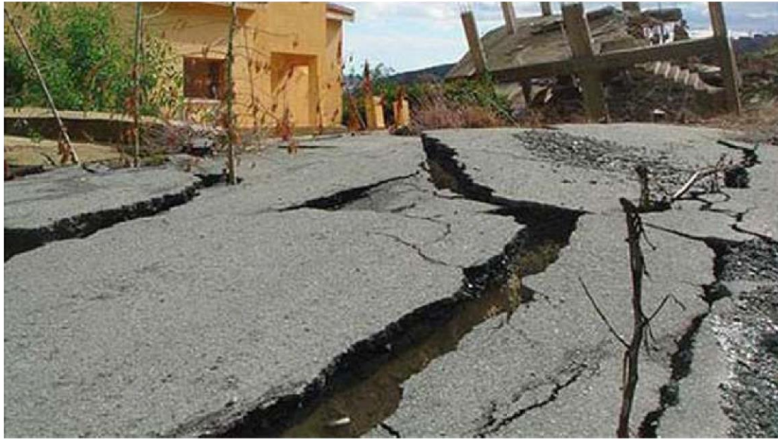
Fig. 3 Landslide in Pissouri area in Cyprus
