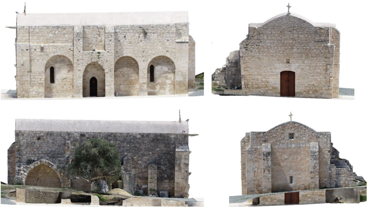
Fig. 5. Elevations of the Church of Panagia Karmiotissa, as taken from the front, back and sides of the Church.
