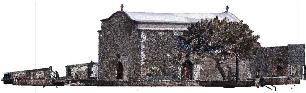
Figure 4: Church 3D model point cloud generated by leica C10 laser scanner
