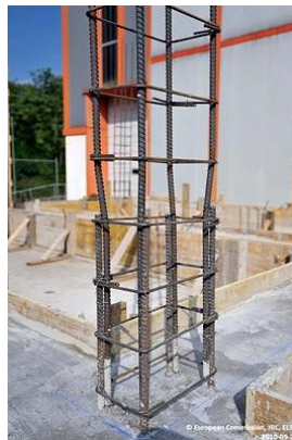
Figure 3.3: Lap-splice of the columns (Poljansek et al. , 2014; Kyriakides et al. , 2015, Poljansek et al. , 2014)
