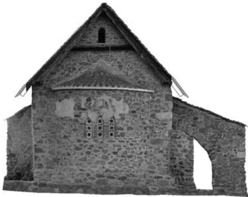
Figure 7: Ortho-mosaic of the eastern facade.
