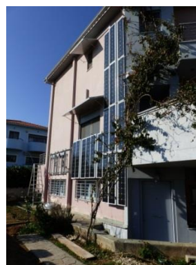
Figure 6: Balconies (left), ventilated façade and canopies (right) in the Greek demo site.
