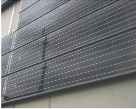
Figure 5: Close-up of the ventilated façade on aluminium element
