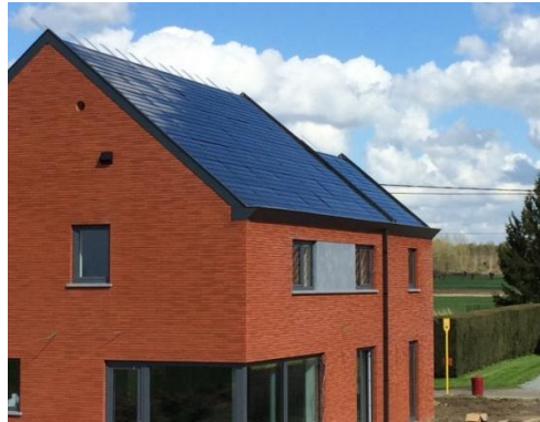
Figure 7: roofing shingles installed in Belgium demo site.
