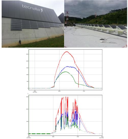
Fig. 4. The retrofitted office building in Zamudio, with the ventilated façade (up left) and skylight (up) generators. Below 2 days of performance (active power) of the 2-generators (blue skylight and green façade) and single inverter and no grid injection (red colored).
