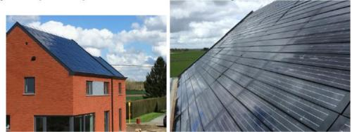
View of demo house in Mons (Belgium) after set-up of BFIRST roofing shingles, May 2016
