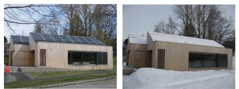
Fig. 1 A building with BIPV on the roof experiencing snow coverage during winter (Living Laboratory, NTNU Gløshaugen Campus, Trondheim, Norway)
